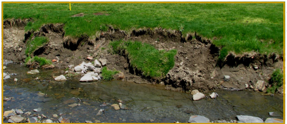
Setbacks and proper stabilization can reduce costly erosion maintenance issues.
