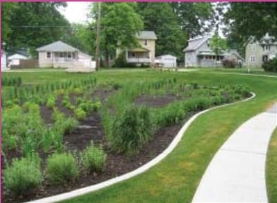
The raingardens at the front door of City Hall will be sized to capture roof runoff from disconnected downspouts the equivalent size of a typical residential roof, demonstrating the use of raingardens to enhance water quality, provide basement flood relief and beautify a neighborhood.
