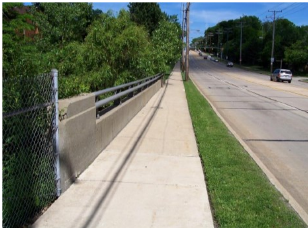
Photo of bridge to monitor from
