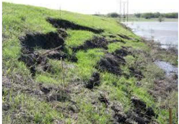
Slumping slope
