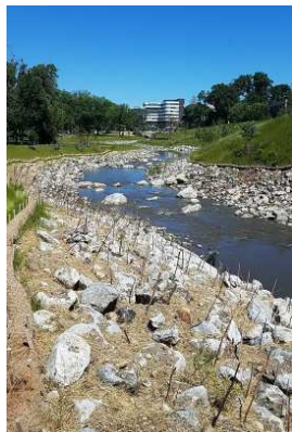
Live Stakes at a restoration project.
