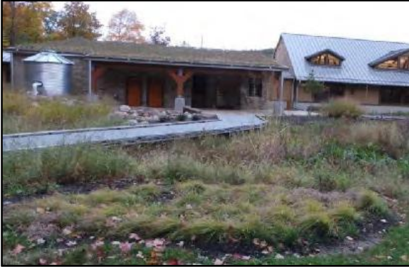
Large cistern (silver tank) capturing stormwater runoff from a green roof at the Cleveland Metroparks West Creek Reservation Watershed Stewardship Center. Credit: Northeast Ohio Regional Sewer District.
