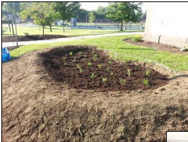
Newly planted rain garden showing shallow, landscaped depression and earthen berm. Credit: Chagrin River Watershed Partners, Inc.
