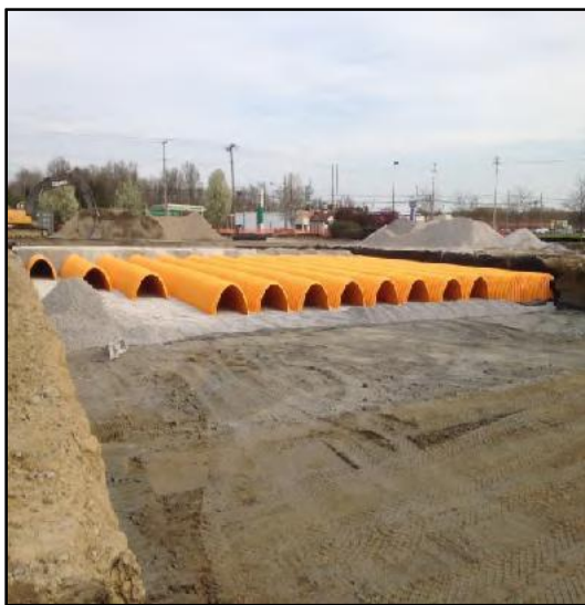
Open-bottom underground detention pipe segments awaiting installation into gravel backfilled storage layer. Credit: StormTech a Division of ADS, Inc.
