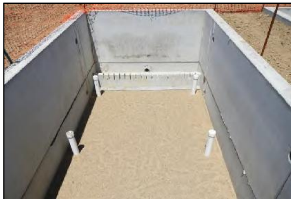
Sand filter chamber showing sand filter bed prior to installation. Credit: Ohio Department of Natural Resources Division of Soil & Water Resources.
