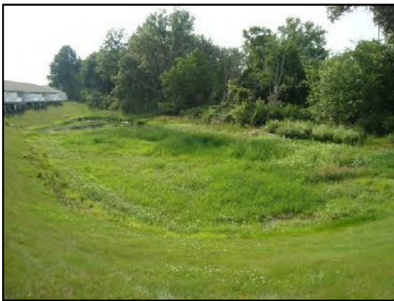
Well maintained dry detention basin. Forebay in the background. Main pool area receives periodic mowing to maintain vegetation. Credit: Cuyahoga Soil & Water Conservation District
