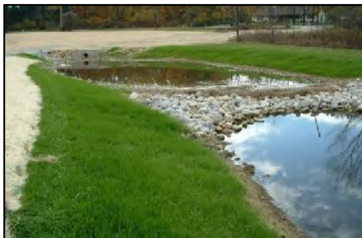
Wet pond containing a forebay pool to capture sediment entering the wet pond from the storm sewer inlet pipe visible in the background. Captured sediment is periodically removed from the forebay area. Credit: Summit Soil & Water Conservation District
